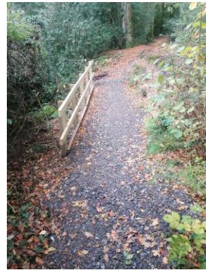
The handrail has been replaced, new drainage and surfacing installed. Steps at the entrance way have been repaired and secured.
